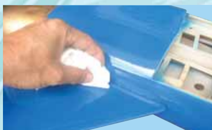
6E - Wipe off the excess epoxy
